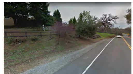
End of the Sidewalk on Alyssum Circle, as seen from Bass Lake Road. Pedestrian & Bicycle facilities are still lacking in the Bass Lake Area
