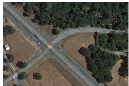
2021 - Green Valley Rd-Deer Valley Rd intersection after 2014 improvements
